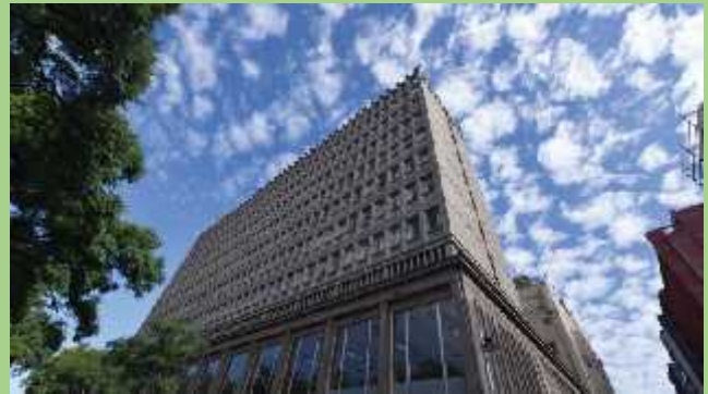
*Existing Building Before Base Building Refurbishment
